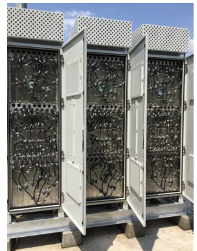
Large outdoor MNCS® system on a building roof
