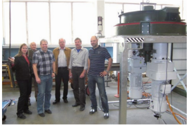
INSTALLATION OF THE FIRST ROTARY JOINT IN THE ROTARY HOUSING WITH TRANSPORT RACK LEFT TO RIGHT: MRS. ZAUZIG, MR. VOGLER, MR. SCHAUBER, MR. GAULE, MR. RIEDEL, MR. GROSS
